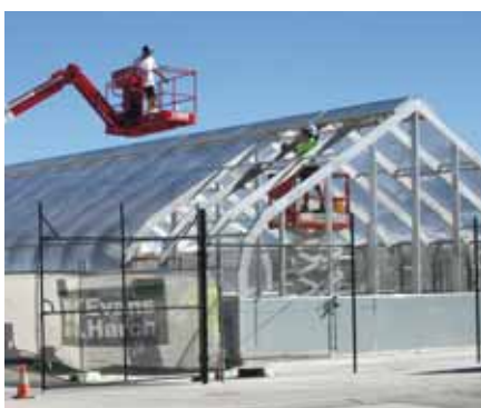
■ Workers construct the CSIRO glasshouse at USC.
